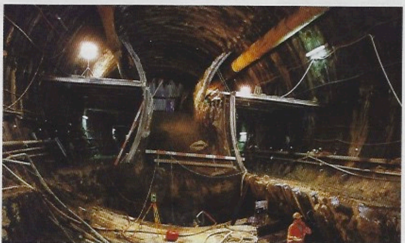
Below: Excavation in the Diebis soft ground section
