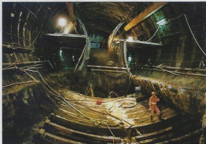
Above: Sequential excavation through the Diebis soft ground section
